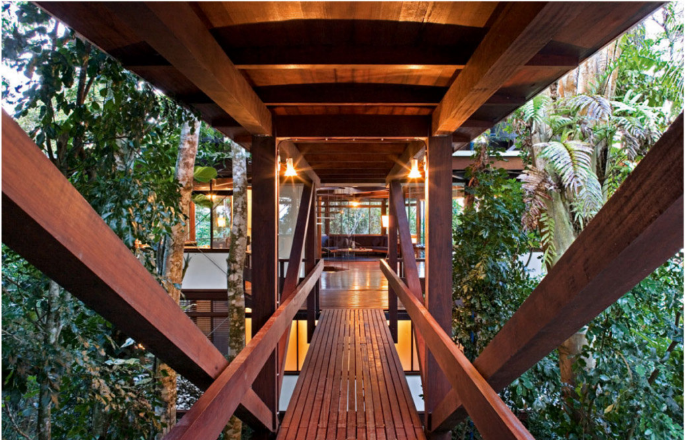
The architect Marcos Acayaba refurbished his own home in Sao Paulo in 2005, redesigning the access bridge to incorporate a new system to cope with the frequent tropical rains. The careful use of natural and local materials makes the house a jewel in the lush setting of the Brazilian jungle / © Leonardo Finott
