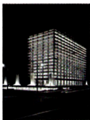
1965 The Department of Water and Power building downtown, by A.C. Martin and Associates
